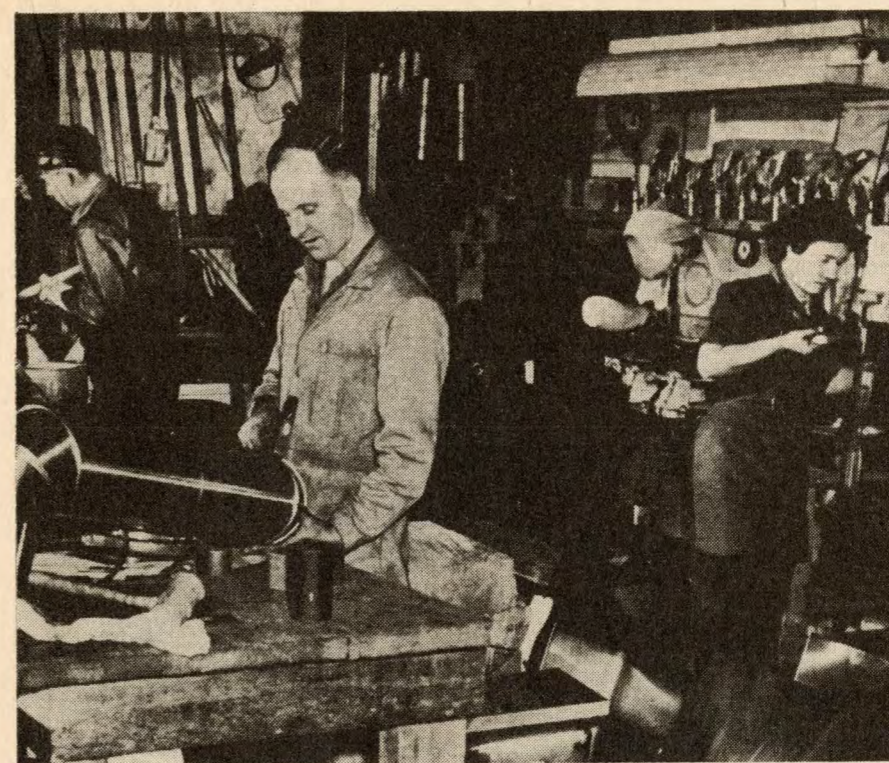
Women found employment during wartime in the sheet metal shop at the shipyards.
