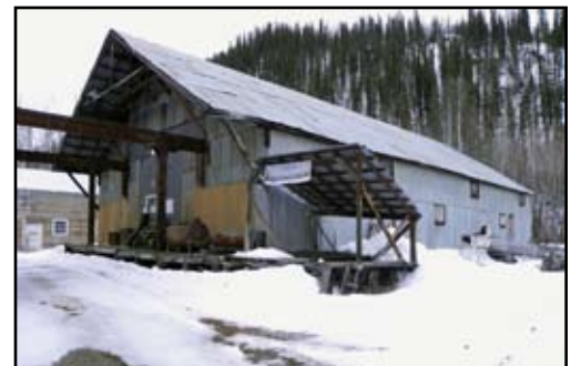
Abandoned and boarded shut building inside Bear Creek Compound.
