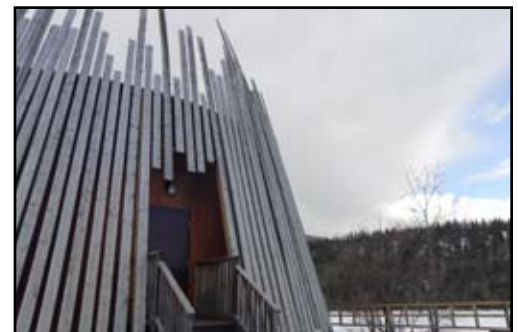
Contemporary design section of the Cultural Centre.
