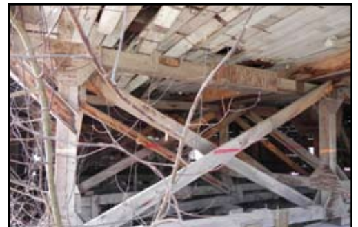
Temporary internal support structure to maintain building shape.
