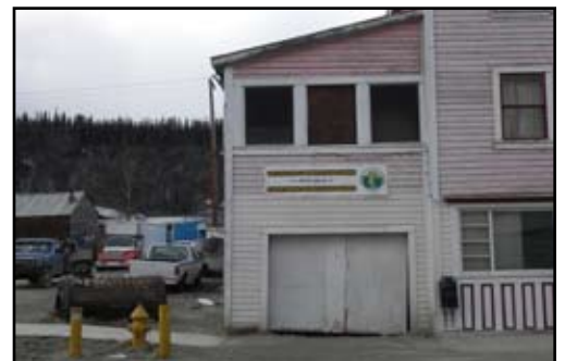
Garage of the Westminster Hotel on 3rd Ave. between Princess & Queen across from SOVA.
