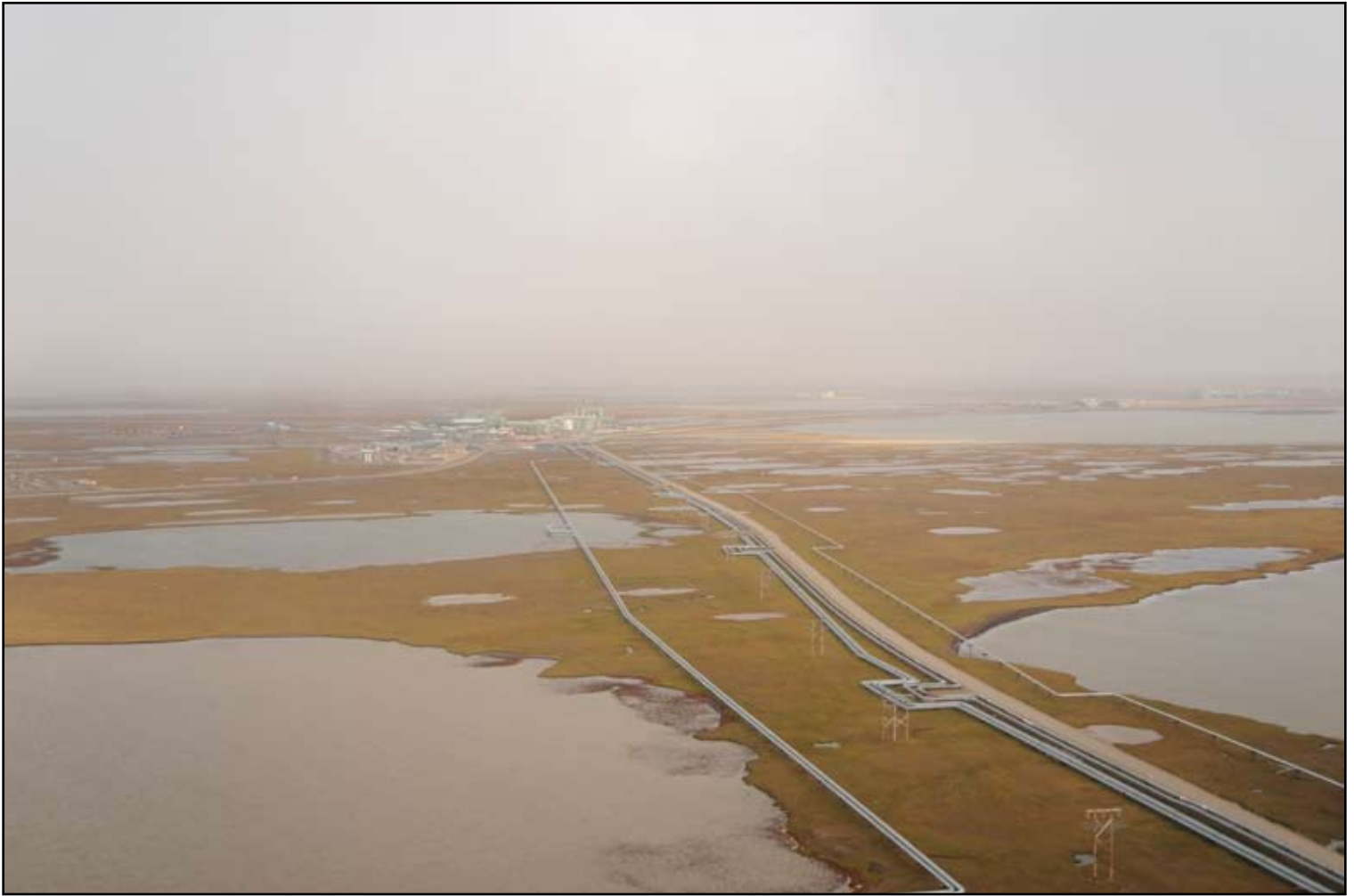
TRANS-ALASKAN PIPELINE: Prudhoe Bay, North Slope, Alaska
